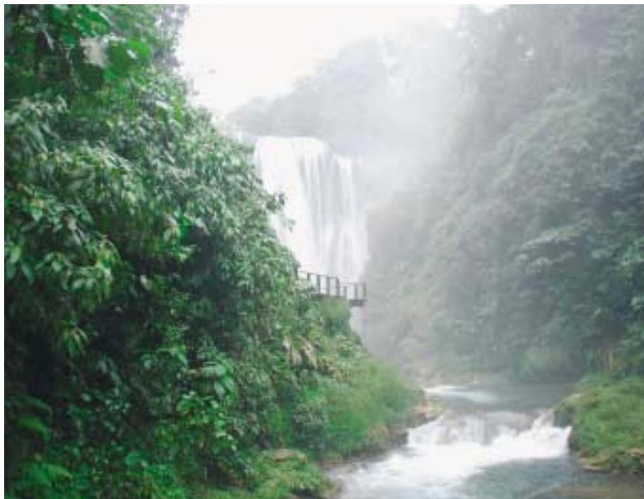
Figure 7–3 In 2005, the Rio Blanco Small Hydroelectric Project in Honduras was registered as the first Finnish Clean Development Mechanism project by the CDM Executive Board. Water flows to the turbines through an underground intake pipe; thus environmental changes in the river channel have been minimised. The waterfalls upstream of the powerplant will remain at their natural state. (Photos: Markku Nurmi).
